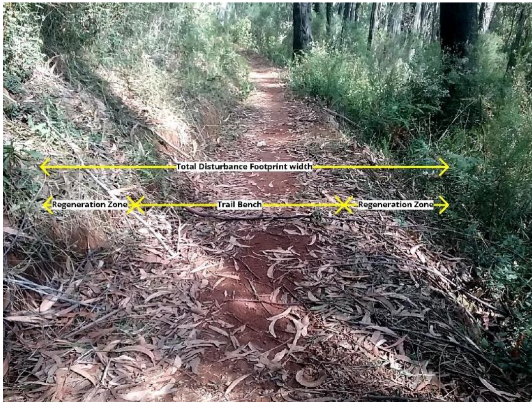
Figure 8-10 Typical trail construction corridor scenario showing the trail bench and temporarily disturbed areas that have regenerated with native vegetation, Yarra State Forest Warburton.
